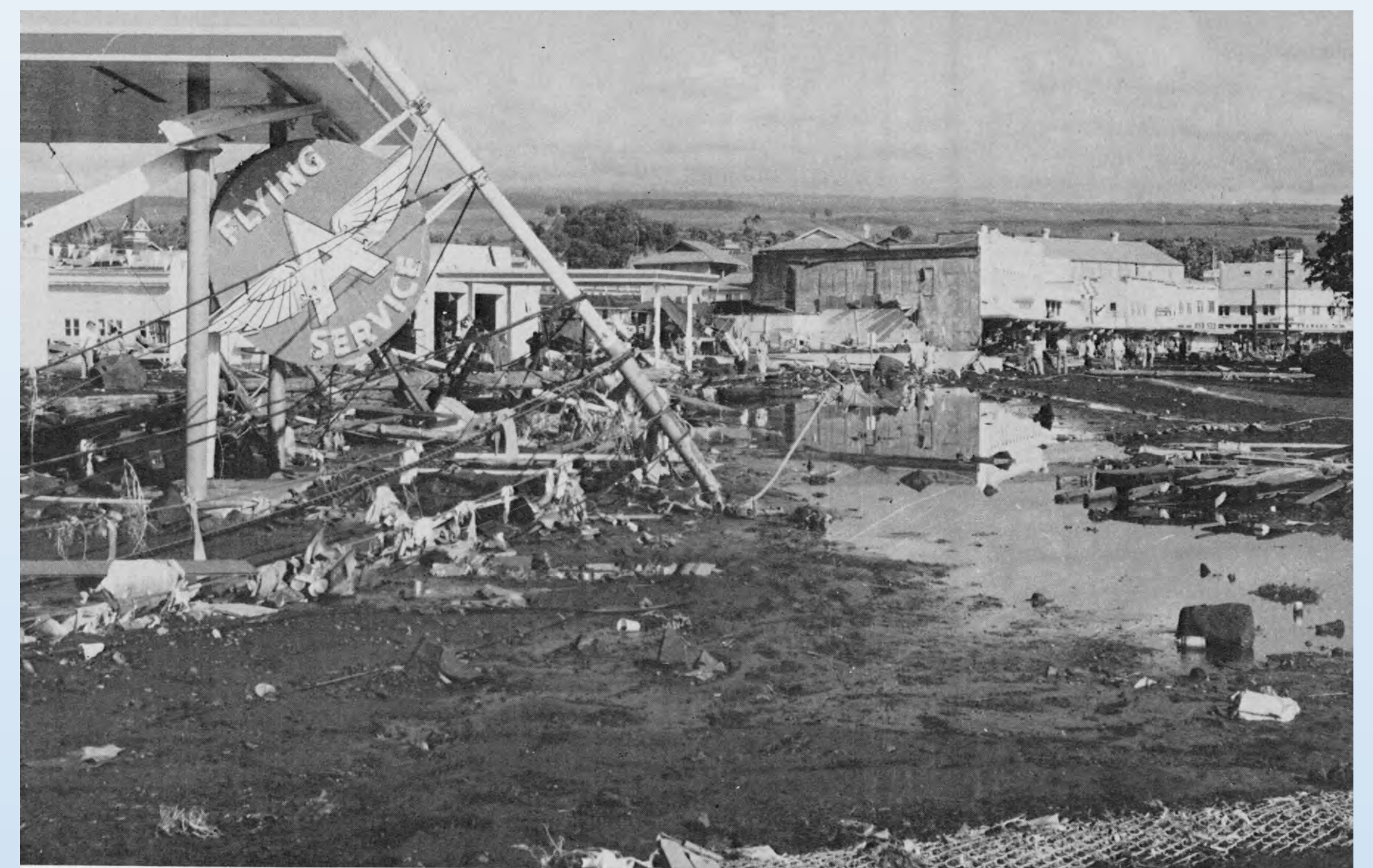
Kamehameha Avenue from the Waiakea side of Ponahawai Intersection after the May 1960, tsunami
