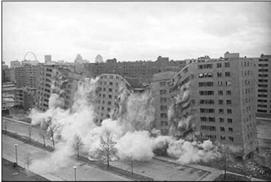
(Implosions commence – note Gateway Arch in the background)
